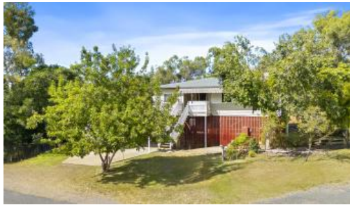
190 Barmoya Road, The Caves
